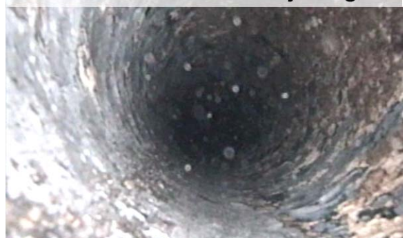
10-in domestic water line at Davis Dam after water jetting.
