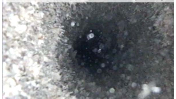
10-in domestic water line at Davis Dam after water jetting.
